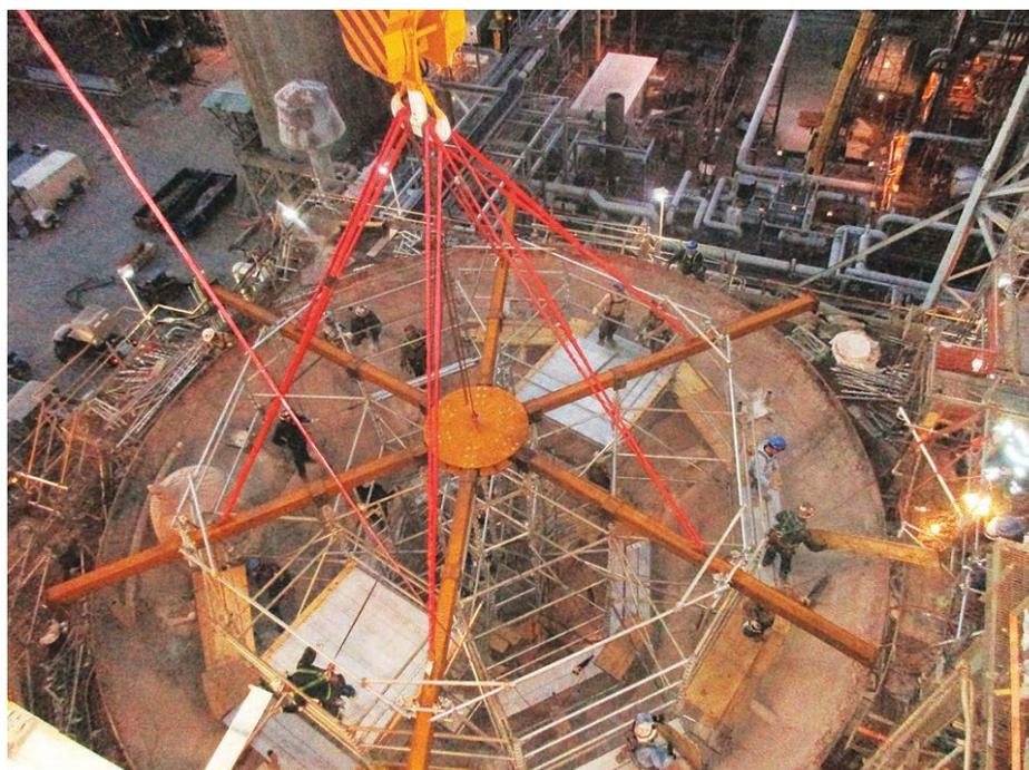
Excel designed the lifting device so the lifting points could be moved and adjusted to fit future lifting applications. The company did not want a "one-and-done" lifting device that would only be cut up for scrap metal once this project was over. With the
