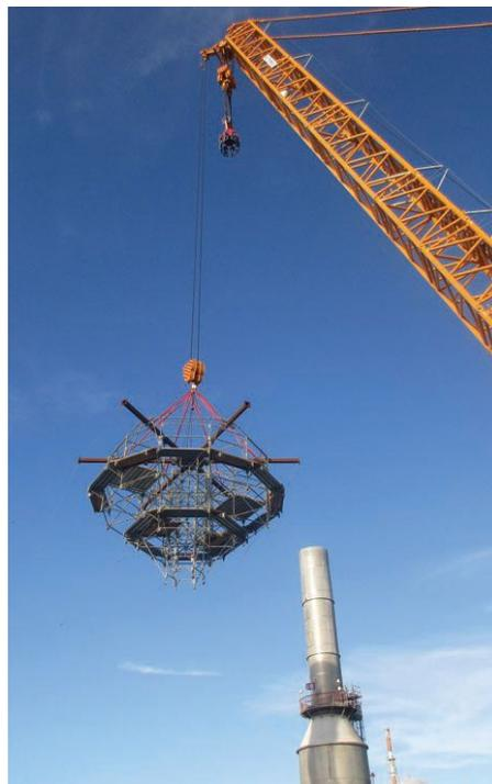
lengths to fit into the cone section. In a short while, Deltak had the lifting device fabricated and load-tested. Once the lifting device arrived on the jobsite, a small crew assembled the lifting device and attached it to the pre-built scaffold. All work was done during straight-time hours, which helped to reduce the cost of the project.
